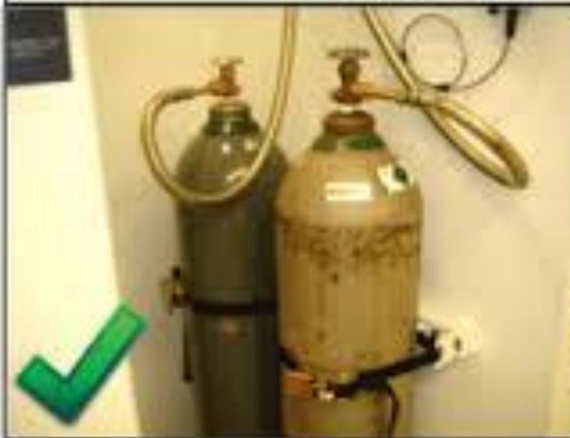
Secure gases \frac{3}{4} of the way up on the tank
